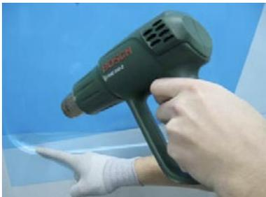
Heat up the material to a temperature between 50 – 60°C. First, you will see some wrinkles on the surface. The film will flatten out afterwards. Start with the deepest corrugation at first!
